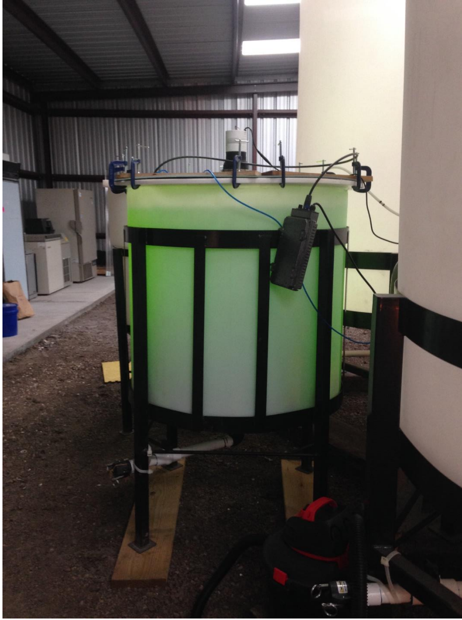
C1B: Inda-gro test tank
